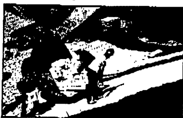
Beveled edges make Armorloc® easy to install by hand, even on difficult to reach sites where pre-assembled mat systems cannot be used.
